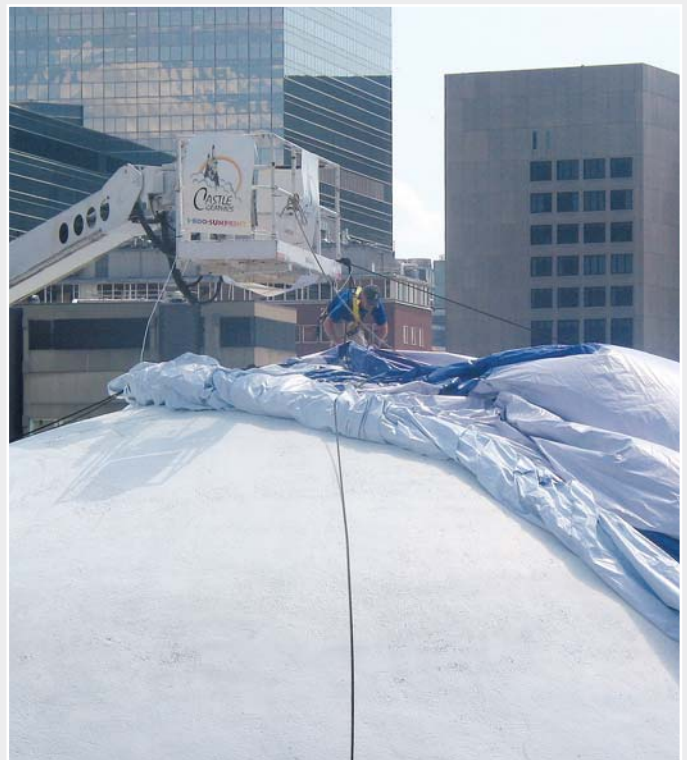
Unravelling the huge plane onto the dome.
