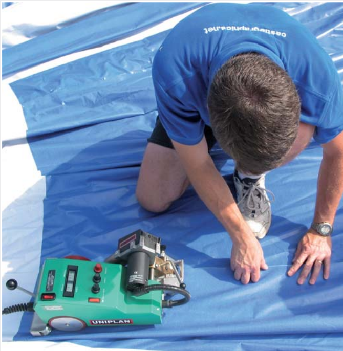
Joining the quadrants with the UNIPLAN E.
