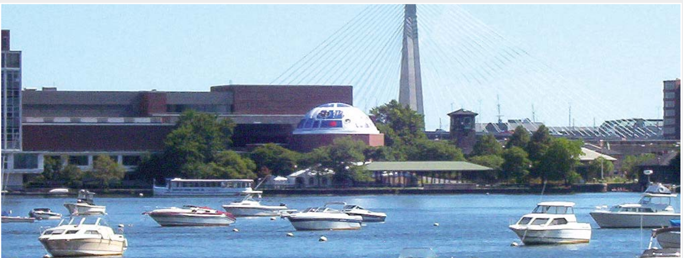
The newly covered dome of Boston's MoS is an actual head turner.
