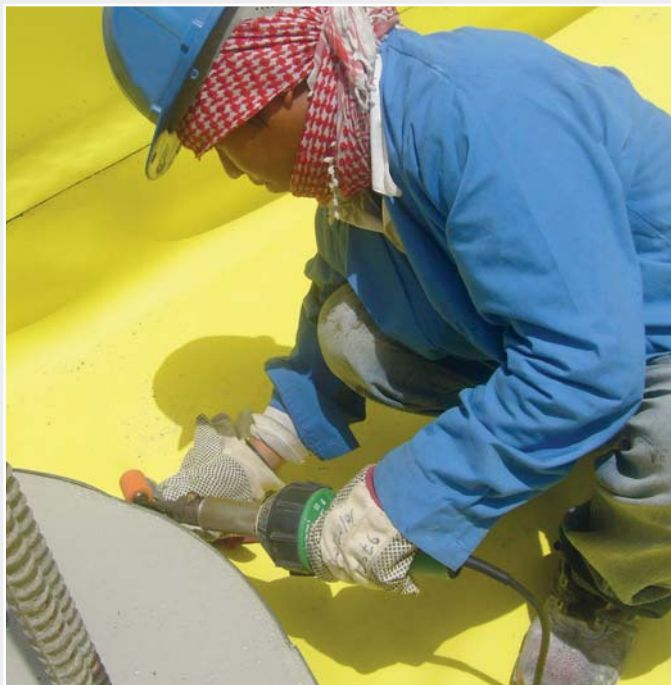
Welding poorly-accessible areas with the hot-air tool TRIAC S and pressure roller.
