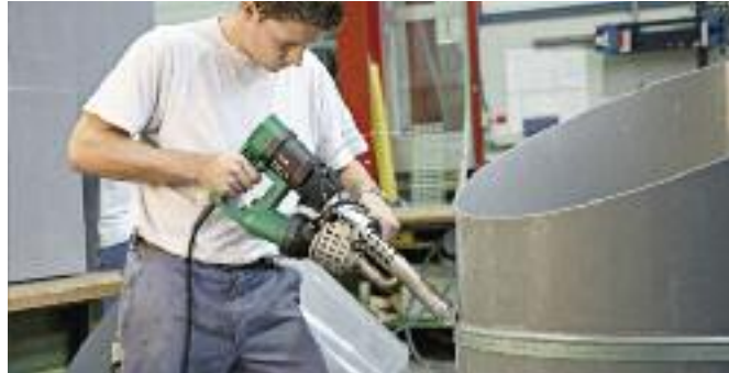
FUSION 3C during the welding of a V-seam.
