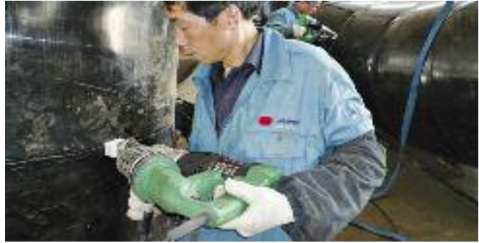
The FUSION 2 in operation during container construction in China.
