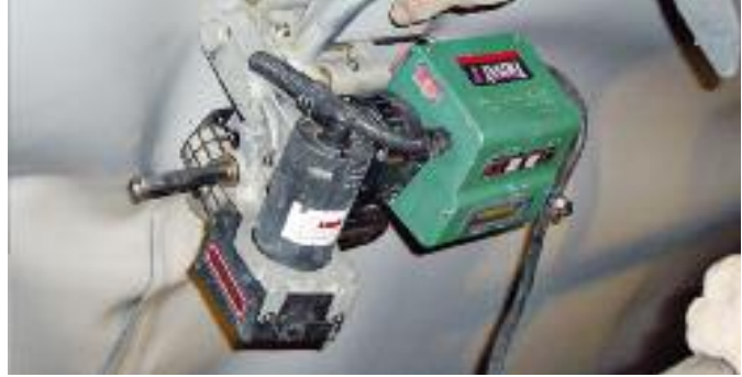
TWINNY T, with convenient cross-handle, at work overhead welding in a tunnel.
