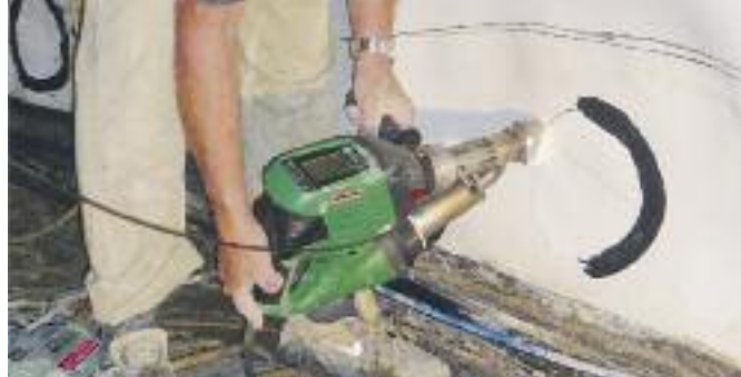
The robust WELDPLAST S2 welding a patch in a tunneling application.
