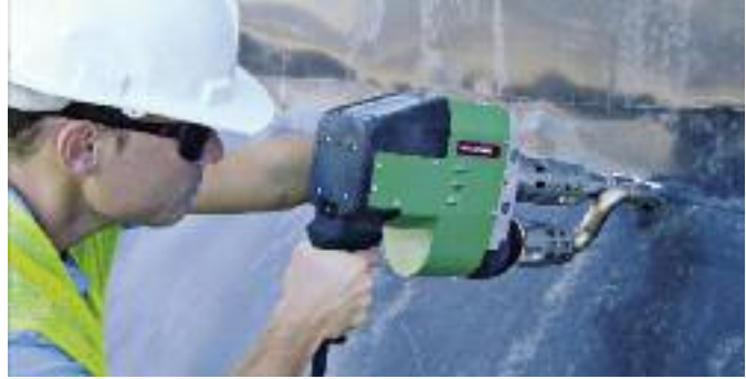
The powerful WELDPLAST S4 at work.
