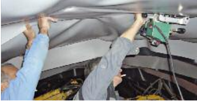
Comet operating in the tunnel ...
