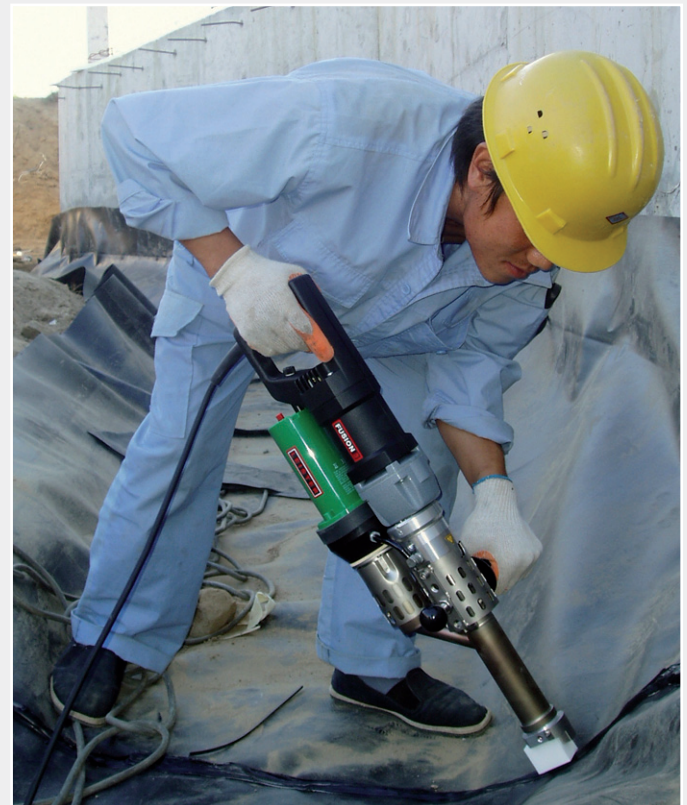
Extruding the sealing sheets on uneven subsurface with the FUSION 3 hand extruder.
