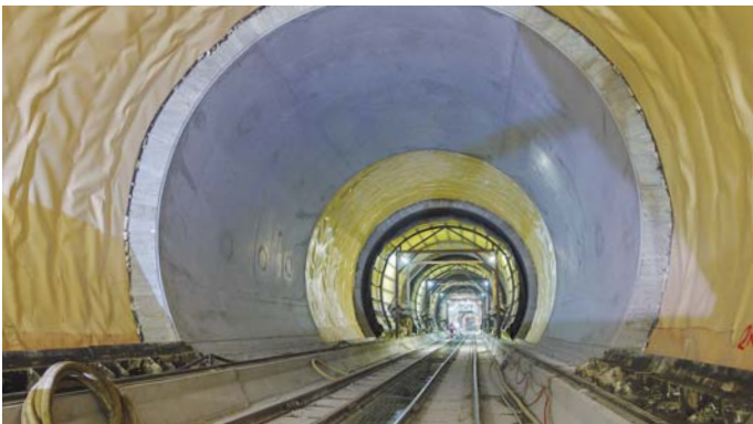
The longest railway tunnel in the world, Switzerland
