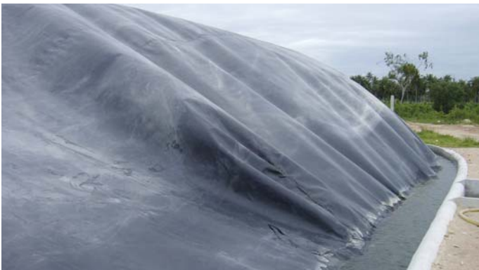
Gas extraction plant in Austria
