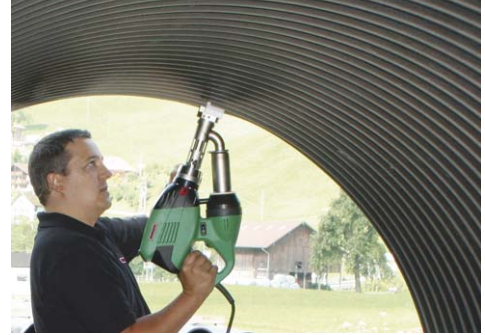
The handy WELDPLAST S2 welding vertically.
