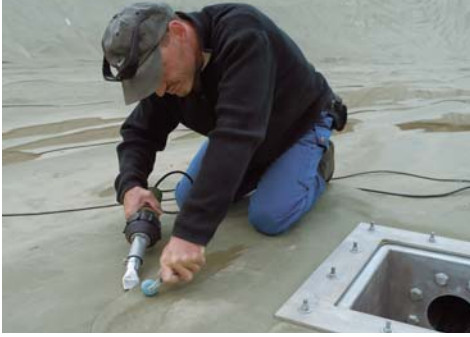
Welding connections using TRIAC PID with push-fit wide slot nozzle.
