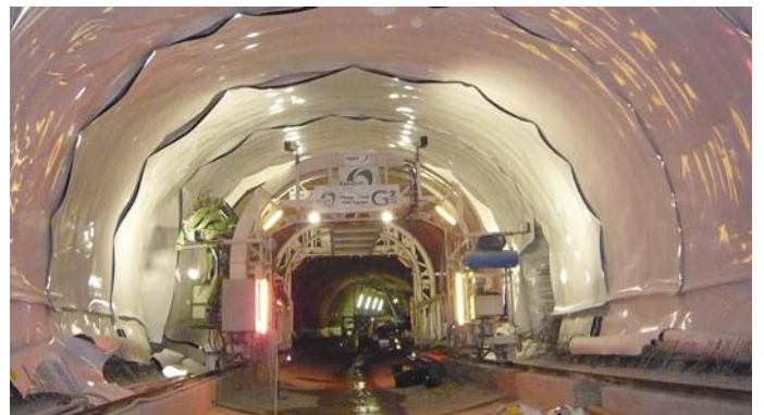
Tunnel construction in Germany
