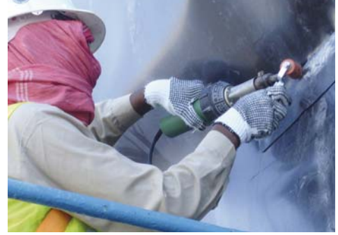
Welding a patch with TRIAC PID on a building site in Dubai.
