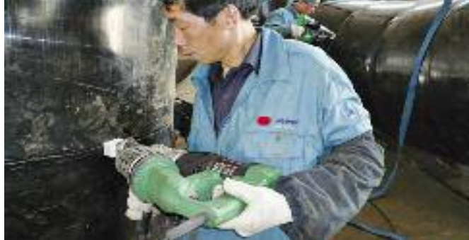
The FUSION 2 in operation during container construction in China.
