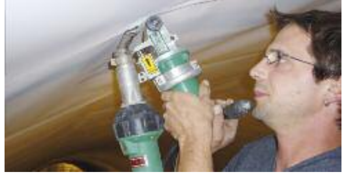
Overhead welding made easy with the TRIAC DRIVE S.
