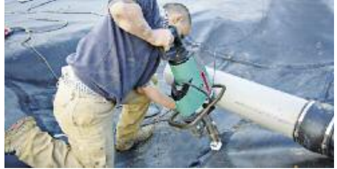
WELDPLAST S6 undertaking assembly applications on a landfill site.
