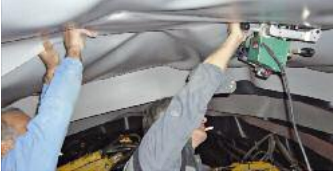
Comet operating in the tunnel ...
